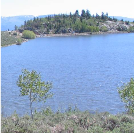
Upper Box Creek Reservoir Dam Outlet
